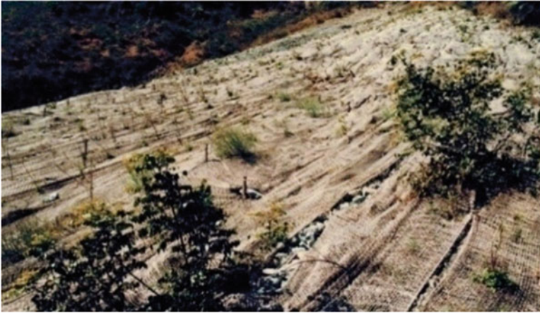
Fig. 17.19 JGT laid over the heap
