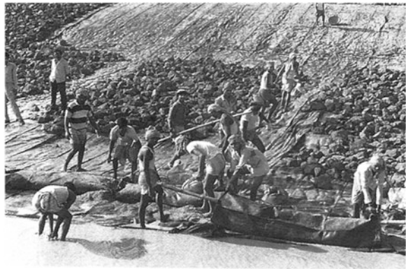
Fig. 17.9 Riprap laying in progress
