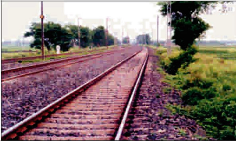
Fig. 17.15 Finished railway track
