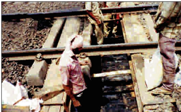
Fig. 17.14 Laying of JGT (woven and nonwoven)
