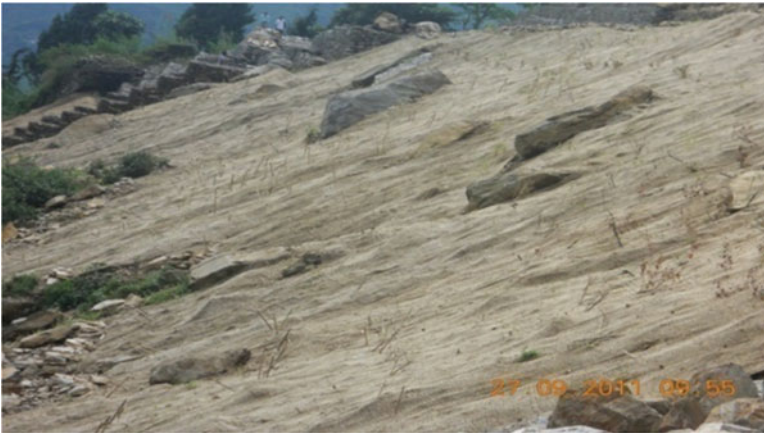
Fig. 17.22 JGT installed over slope
