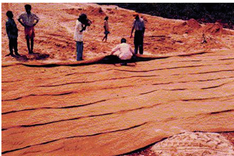
Fig. 17.3 JGT installation in progress
