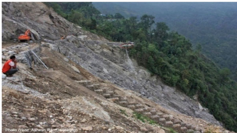
Fig. 17.23 Cascading in progress
