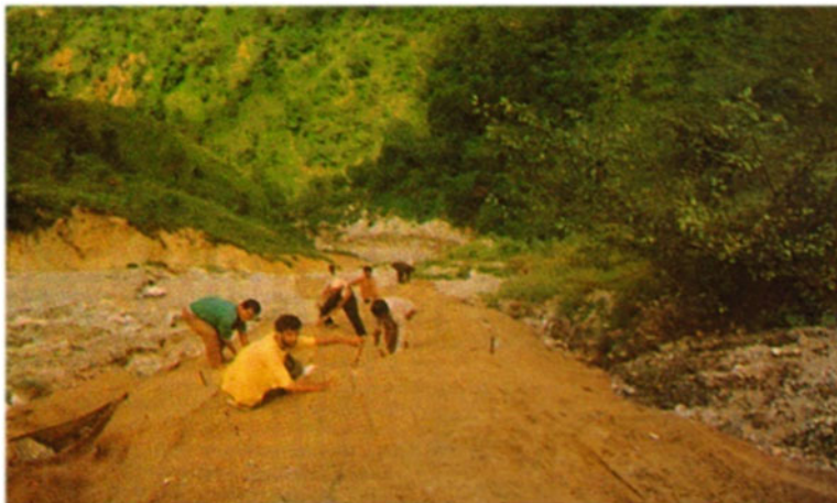
Fig. 17.20 JGT under installation
