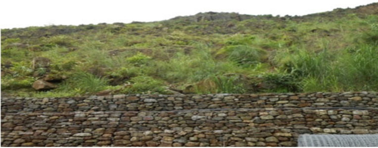
Fig. 17.24 Stabilized slope after reclamation with JGT
